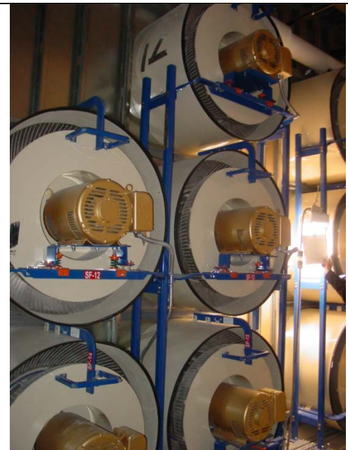
Tall/narrow aspect ratio 78,500 CFM at 6" SP
